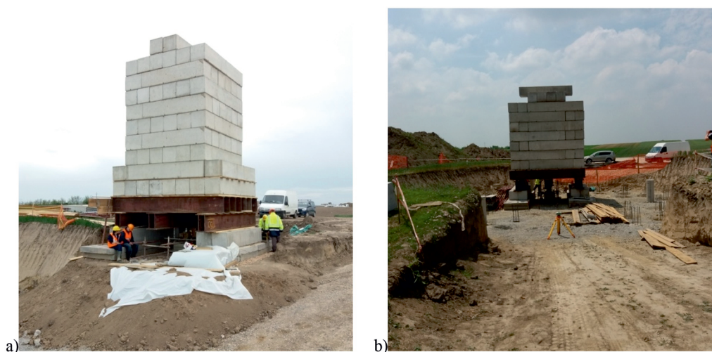
Fig. 1. Created counterweights for conducting in-situ SLT of piles of wind turbines: a) WT 1, b) WT 2
