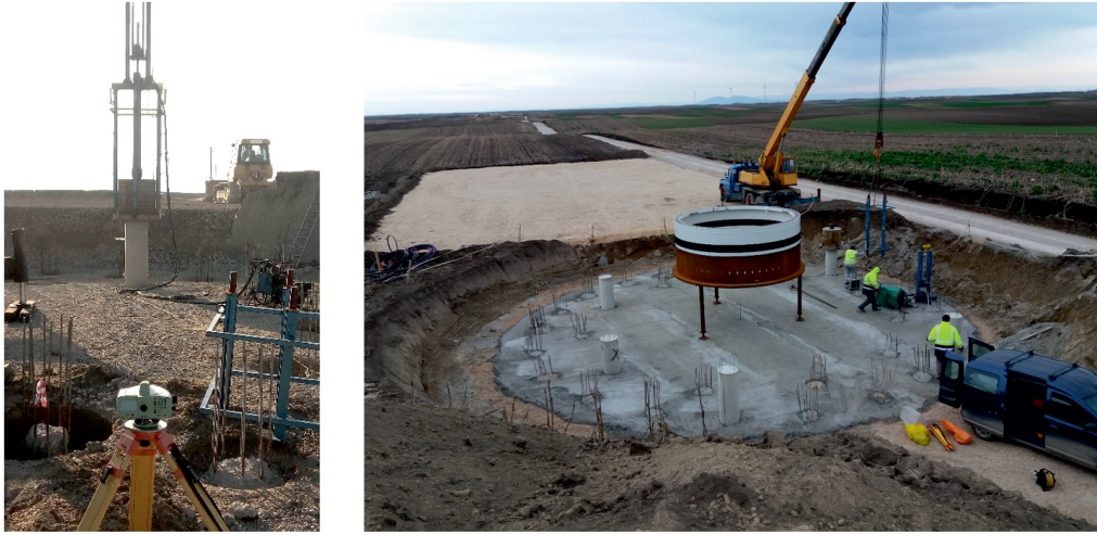
Fig. 2. In-situ tests and equipment for DLTs of wind turbine WT 1 and WT 2 piles
